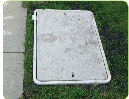
Installation of service box in utility right-of-way.
